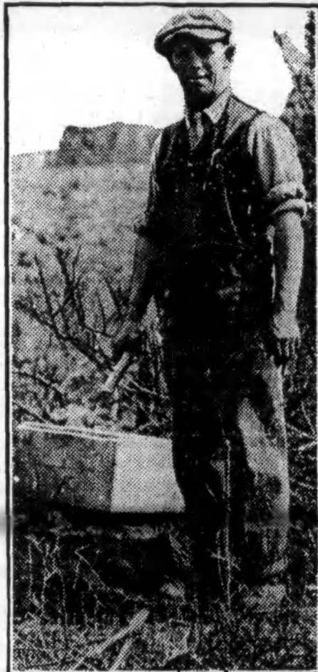
PREPARING A DYNAMITE BLAST.
