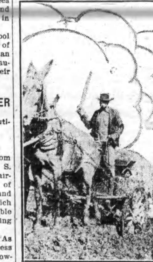
ON AN UNRECONSTRUCTED DIRT ROAD.
