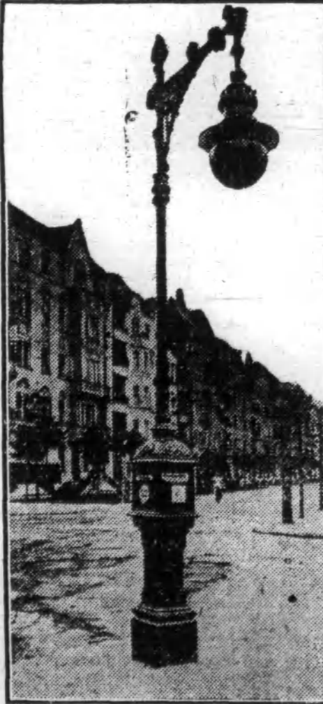
A GERMAN FIRE ALARM BOX.
