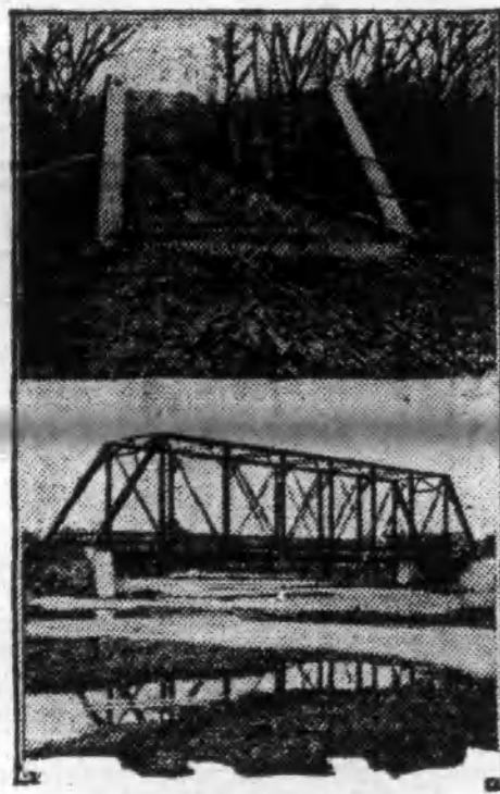
STEEL BRIDGES; LOWER ONE SHOWS CONCRETE ABUTMENTS.
