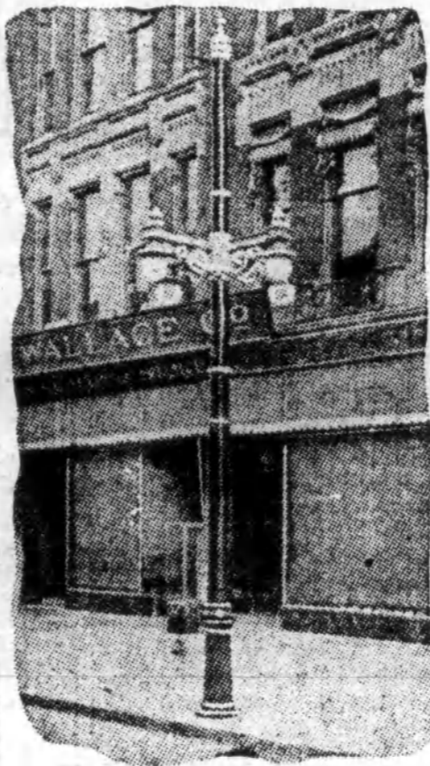
COMBINATION LIGHT AND TROLLEY POLE.
