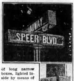
eight candle power incandescent lamps. The light is reflected to the signs from the interior, the letters being on a background of mica.
