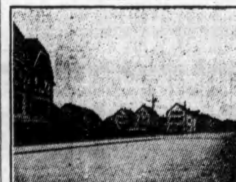
THE RESULT AFTER STREET HAS BEEN TREATED WITH OIL.
