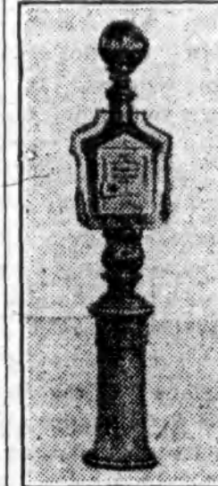
LIGHT ON FIRE ALARM BOX.
