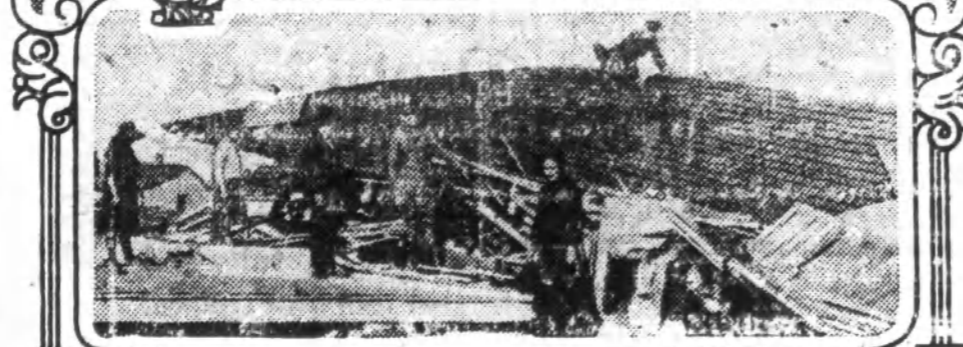
A force pressed into service in the wake of the southern tornado. (Below) Salvation Army workers amid the ruins of La Grange, Ga.
